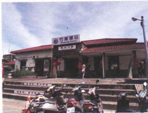
▲ Zhudong Train Station.
